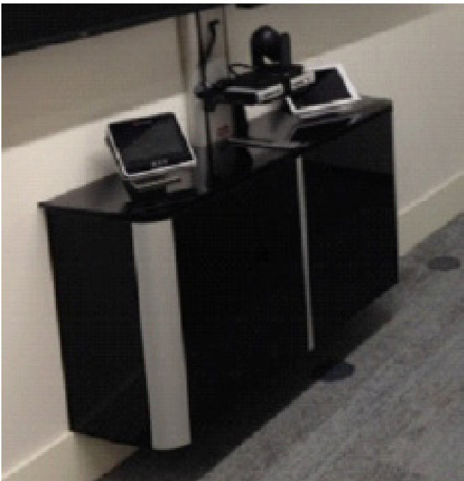
Wall mounted twin 6u vertical rack
