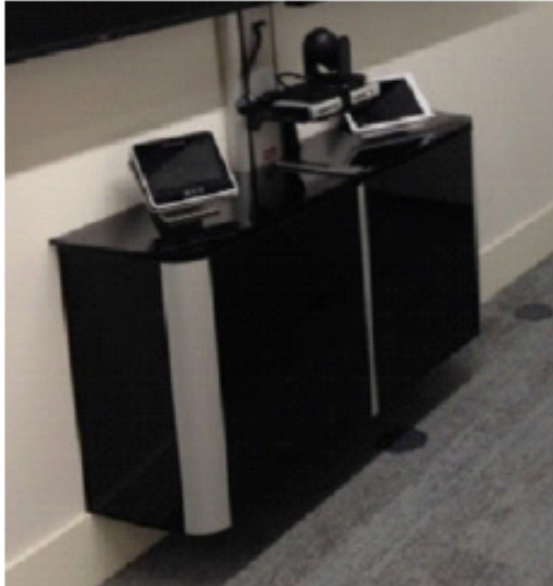
Wall mounted twin 6u vertical rack
